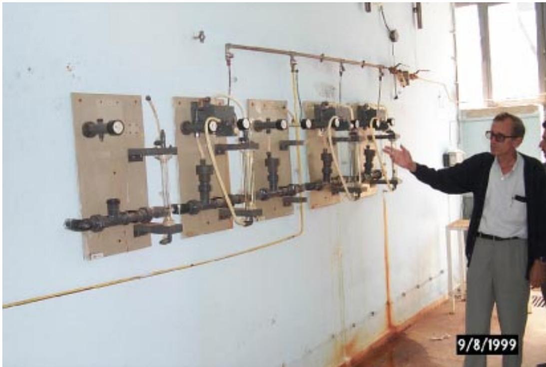
*Figure 18. Damage to Five Chlorine Mixing Units – Yalova WTP*
