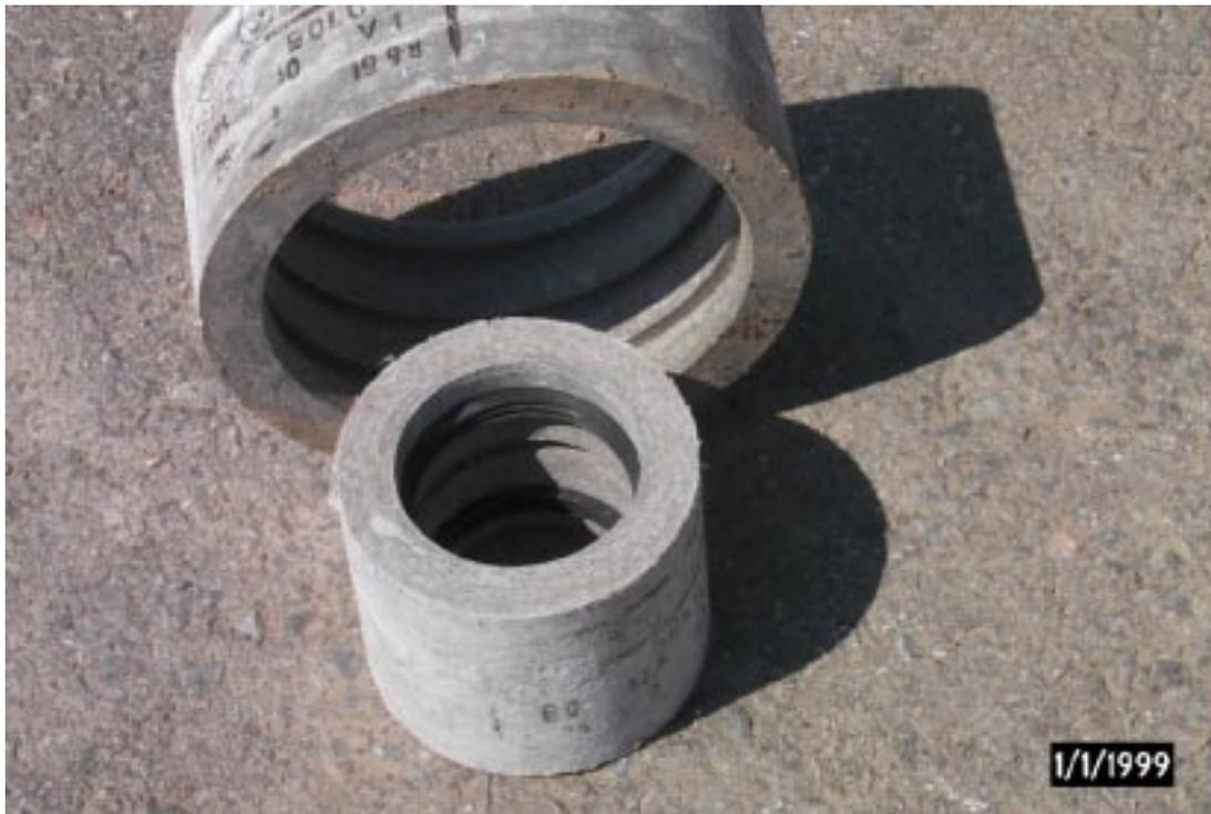
*Figure 10. Typical Rubber Gasket Joint Fitting for AC Pipe, Common to All Water Systems in the Area*
