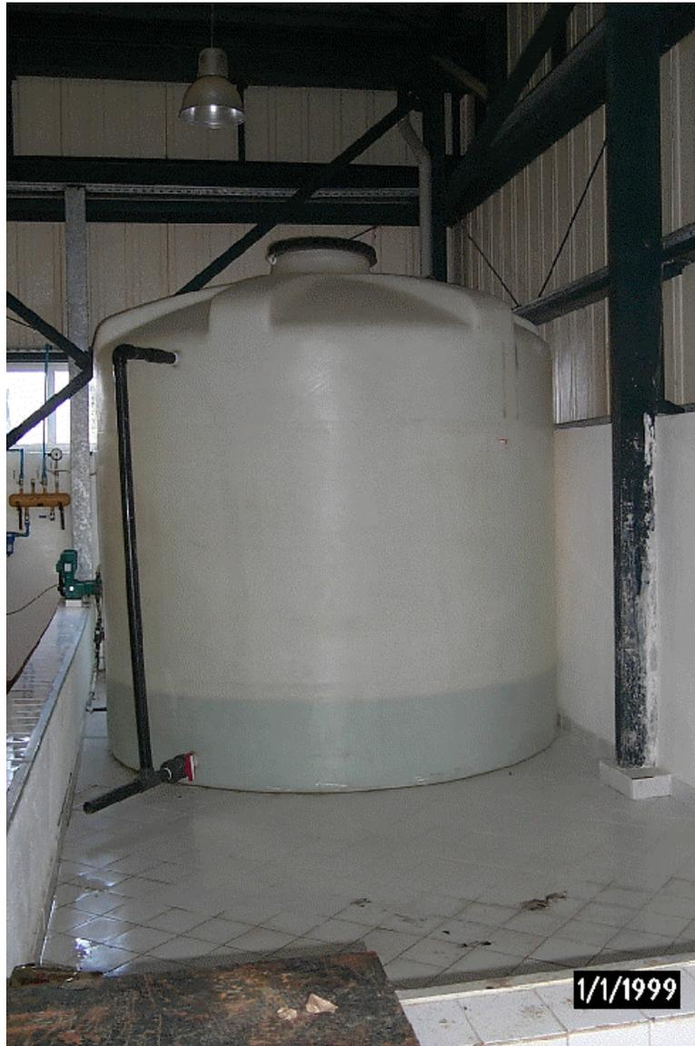
*Figure 7, Unanchored Plastic Tanks – Maltepe WTP*
