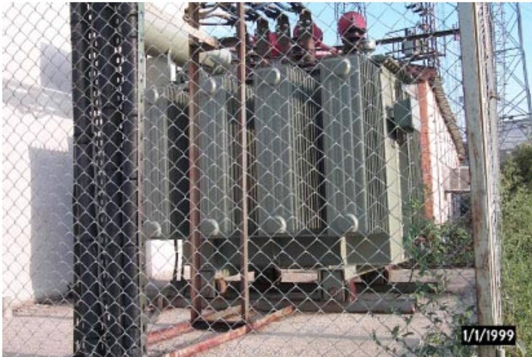
*Figure 9. Unanchored Transformer Serving Maltepe WTP. A Bushing was Damaged.*
