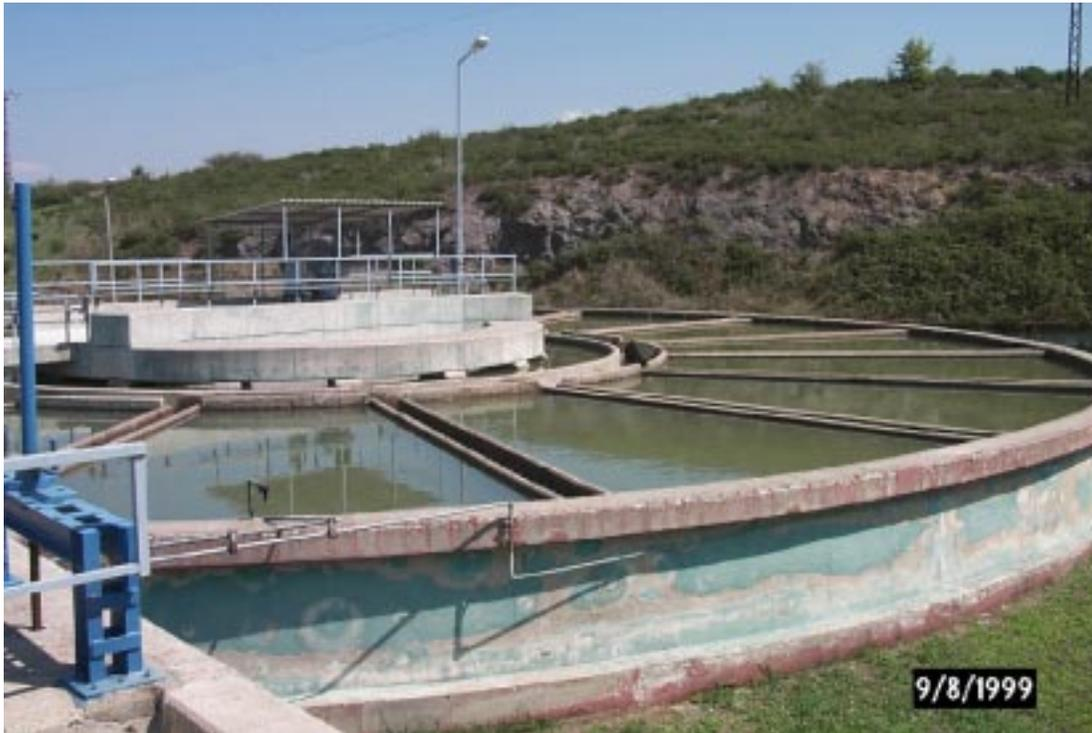
*Figure 19. Clarifiers at Yalova WTP. No Damage to RC Water Troughs or Baffles*
