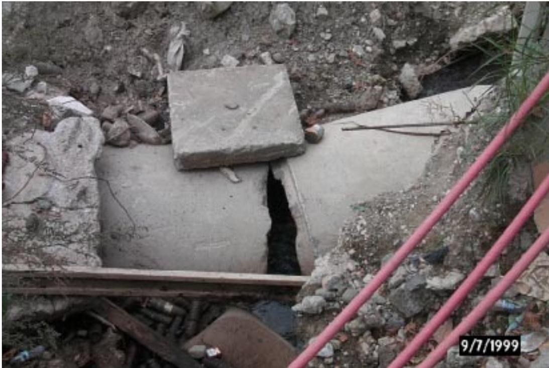
*Figure 15. Broken Sanitary Sewer in Adapazari.*
