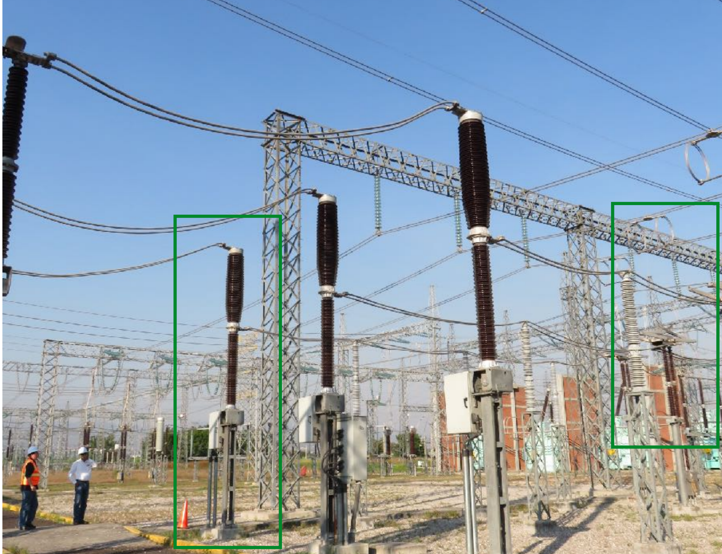
230 kV CBs 3 / 6 collapsed. May have been aggravated by collapse of adjacent Scissor Switches, note the tight slack
