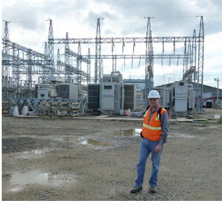
*Figure 4-37. Transformer Banks at Tagajyo Substation, June 14, 2011*
