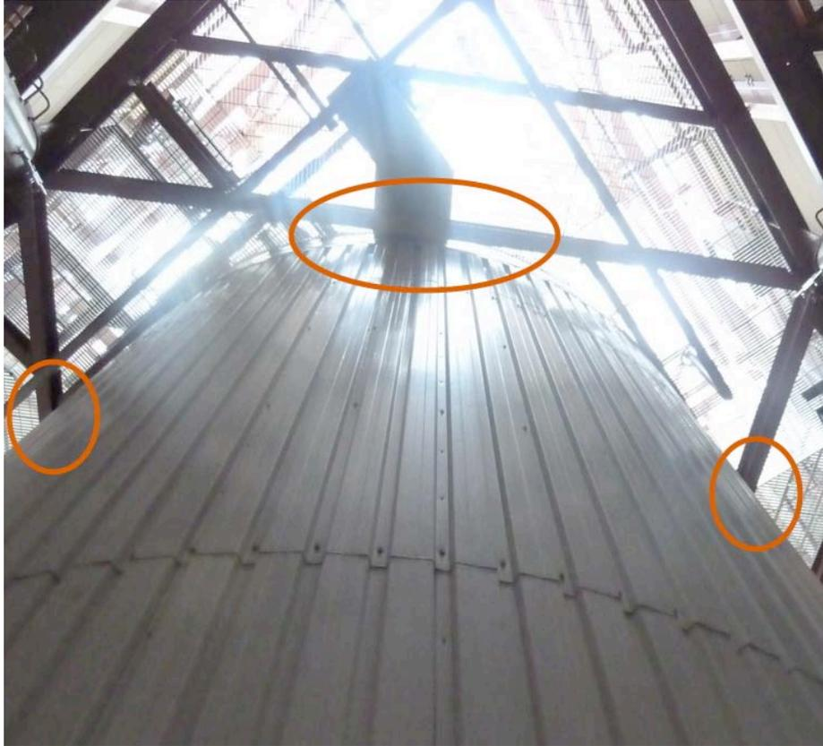
*Figure 4-30. Braces Around Chimney Stack.*
