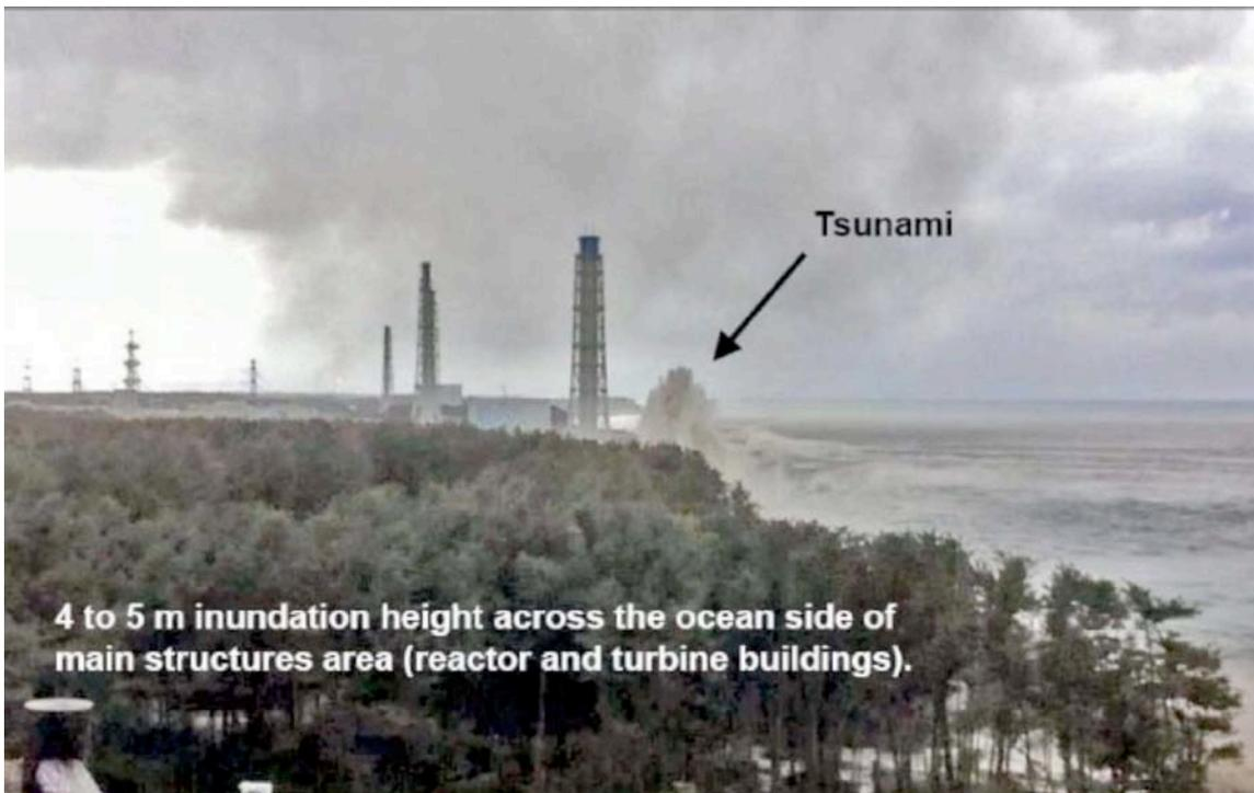
Figure 4-98. Tsunami Impacting Fukushima Daiichi (photo credit John Luxat McMaster)
