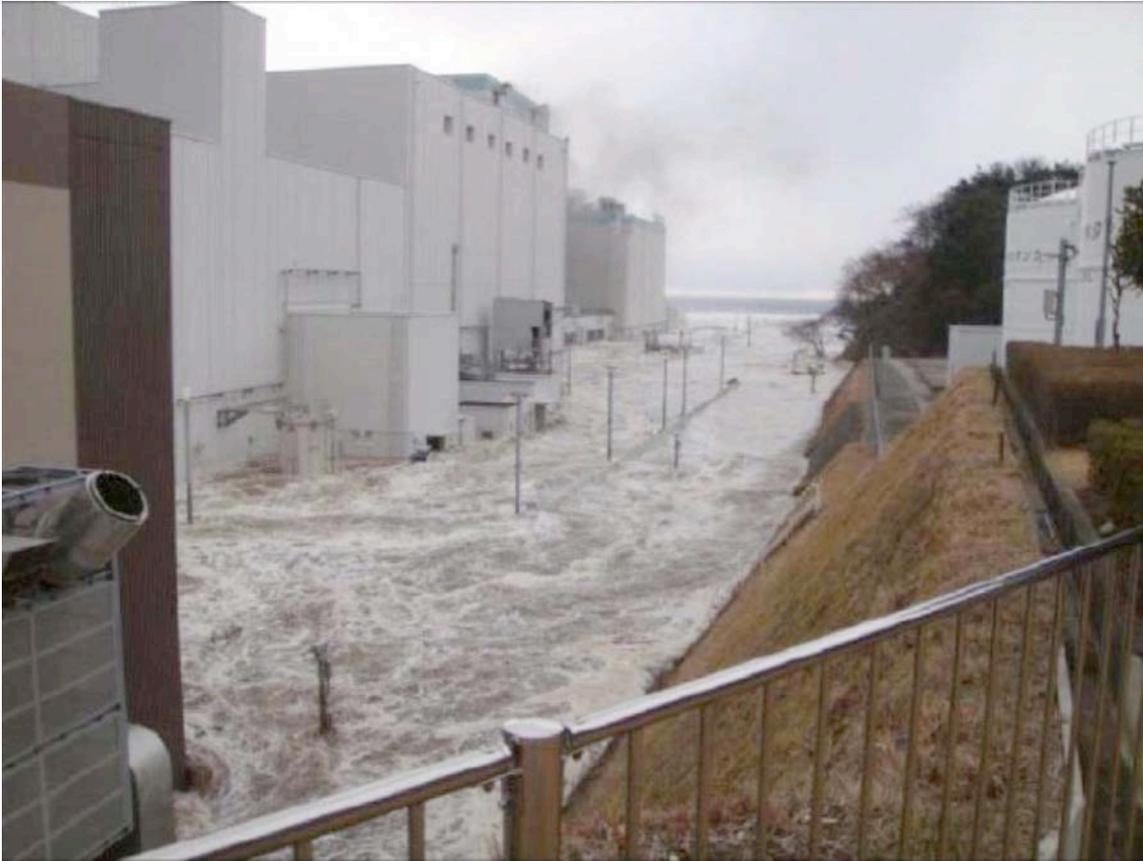
*Figure 4-99. Tsunami Flooding the Salt Water Pump Pits at Fukushima Daiichi (photo credit John Luxat McMaster)*
