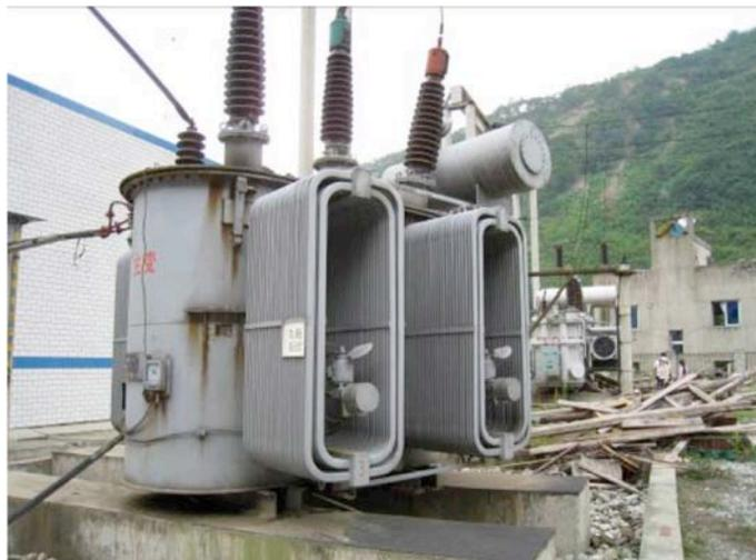
*Figure 5. Skid-Mounted Transformer*
