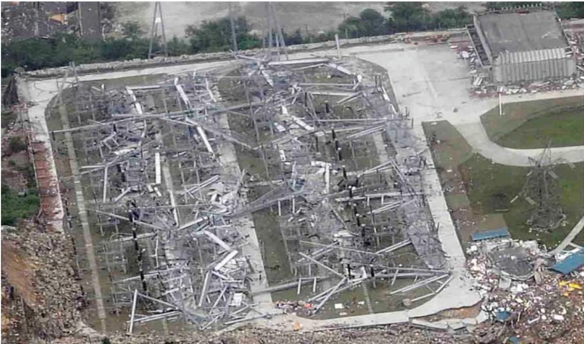
*Figure 9. Destruction to Ertai Shan Substation, 220 kV, Yingzhou*
