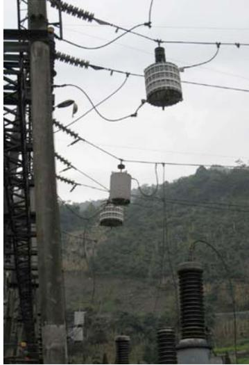
*Figure 8. Hanging Wave Traps and Damage to Bus Connections to PTs*
