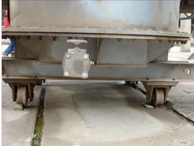
*Figure 3. Wheel-Mounted Transformer*
