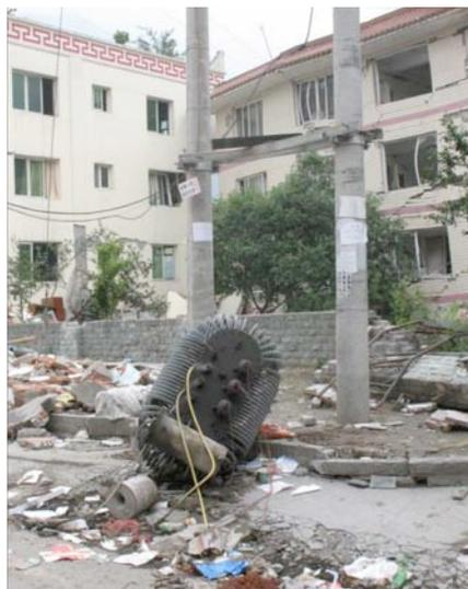
*Figure 13. Fallen Distribution Transformer*
