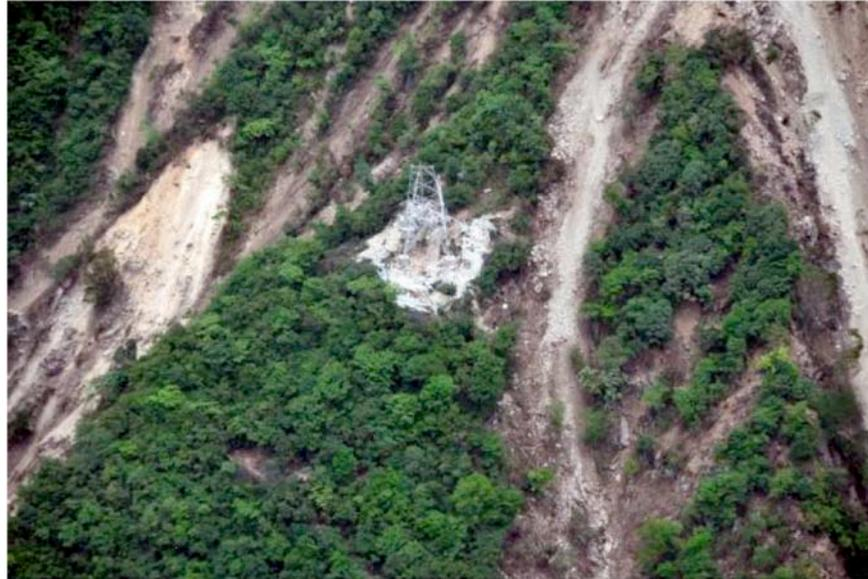
*Figure 10. Collapsed Tower*
