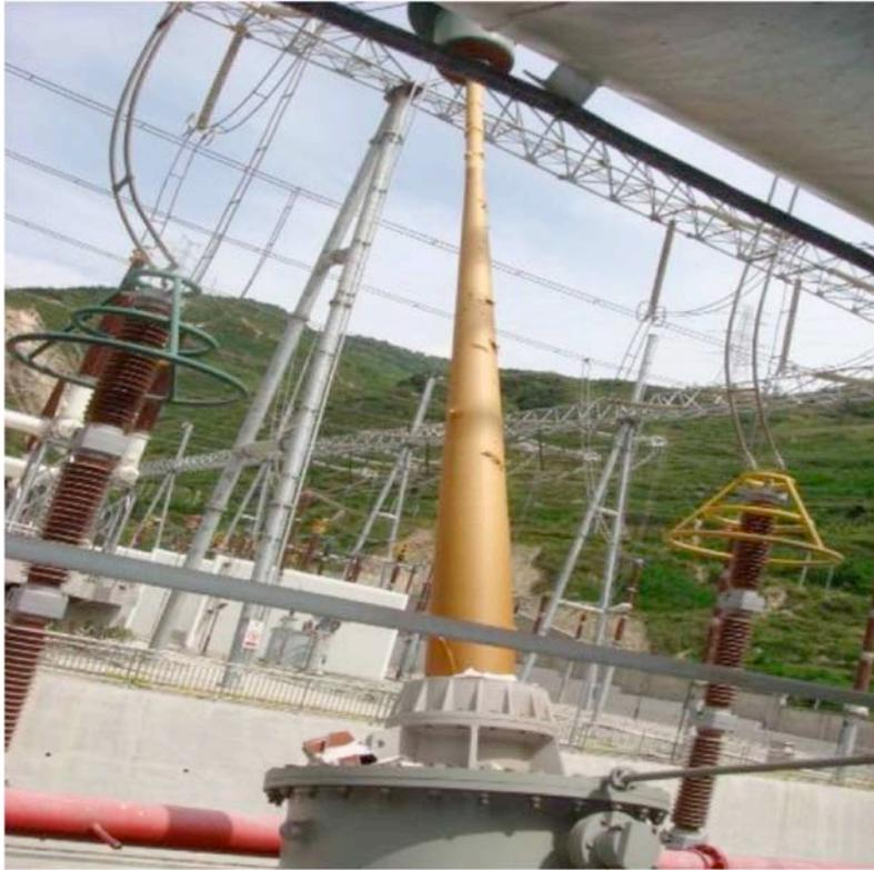
Figure 6. Bushing, 500 kV Transformer
