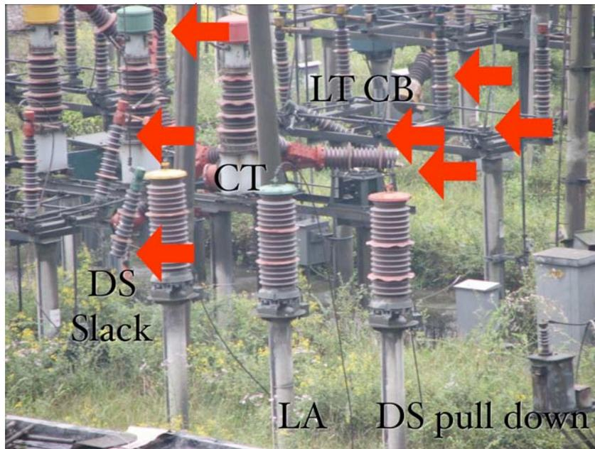
Figure 7. Examples of damage to Yard Equipment, Yingzhou 110 kV Substation
