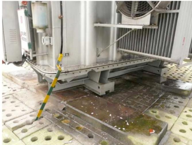
*Figure 4. Skid-Mounted Transformer*
