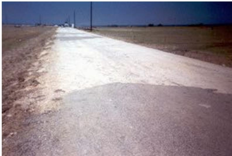
Figure D-6. Typical F5 Tornado Damage (Asphalt). The asphalt surface has been peeled off of this road.
