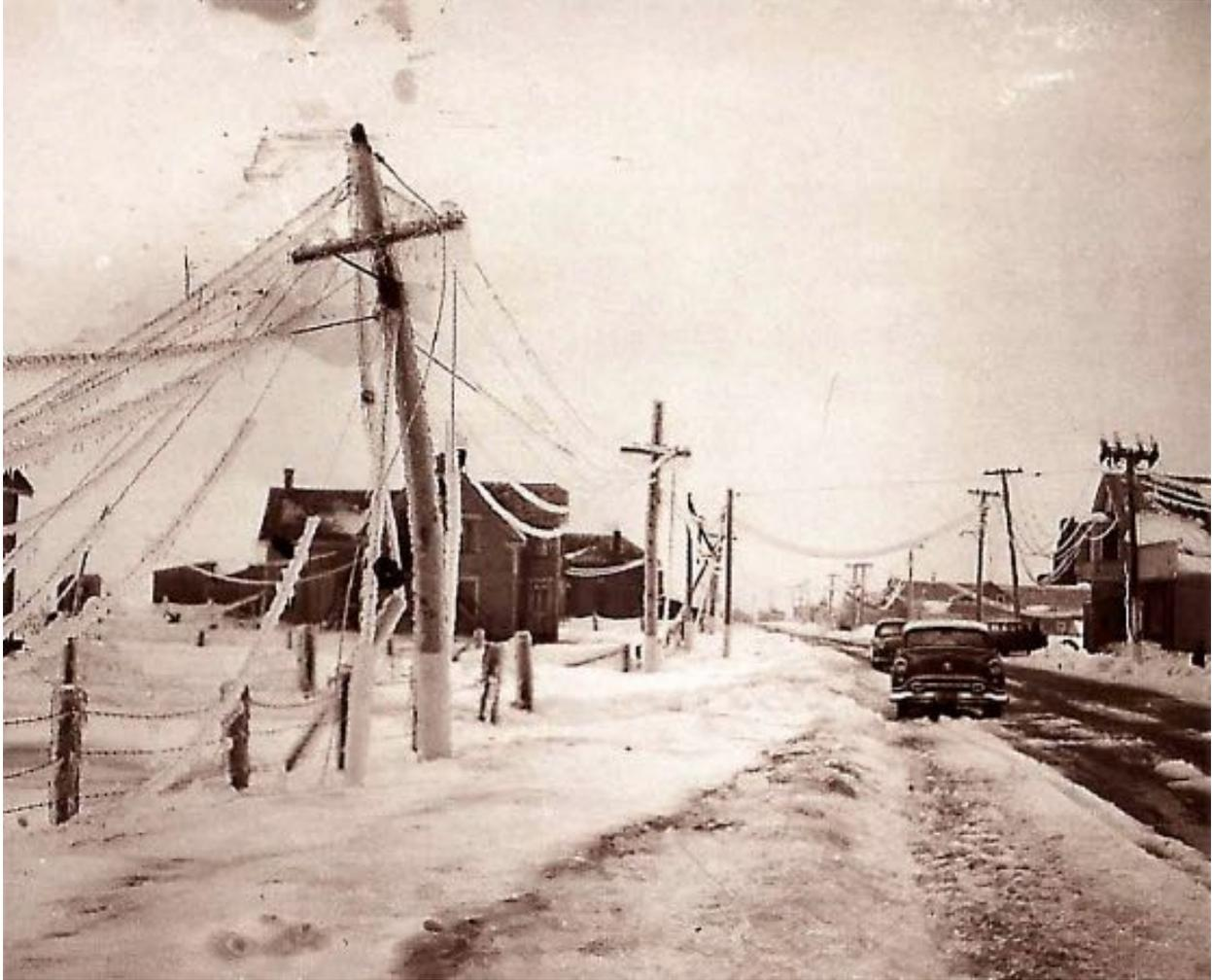
**Figure 5-11. Ice Storm Damage, January 2, 1956**
