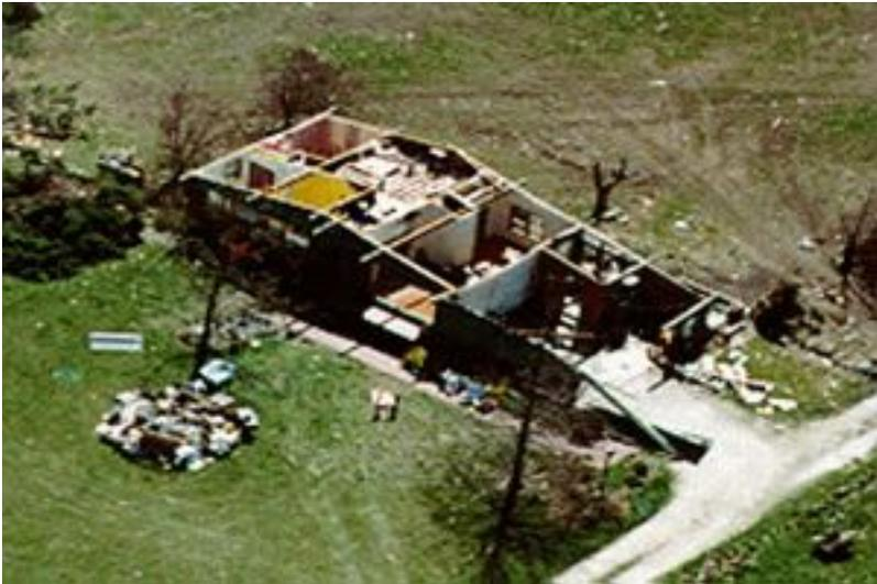
Figure D-3. Typical F2 Tornado Damage. This home is missing its entire roof but the exterior walls remain intact. Some of the stronger hardwood trees remain standing.
