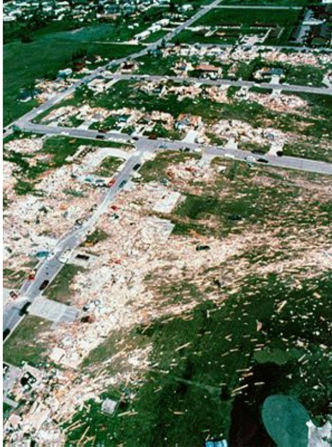
Figure D-7. Typical F5 Tornado Damage (Homes). These homes have been completely removed from their original locations. The debris field has been scattered some distance from their foundation.
