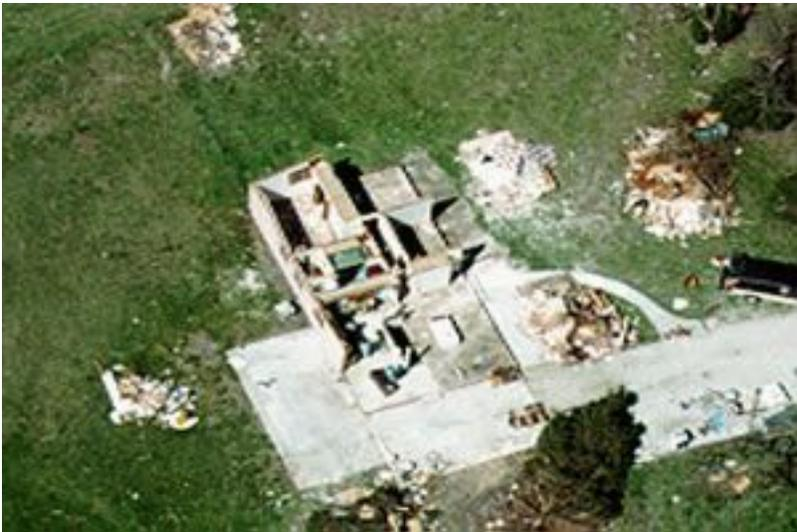
Figure D-4. Typical F3 Tornado Damage. This home is missing the entire roof as well as some of the exterior walls. Trees are blown over or snapped near the base and outbuildings are destroyed.
