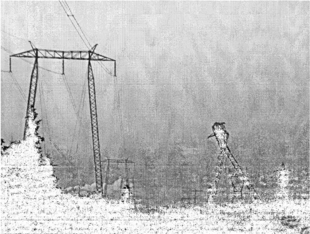
**Figure 5-7. Damaged Tower Type A 301 (right side). Undamaged Tower Type A (left side)**
