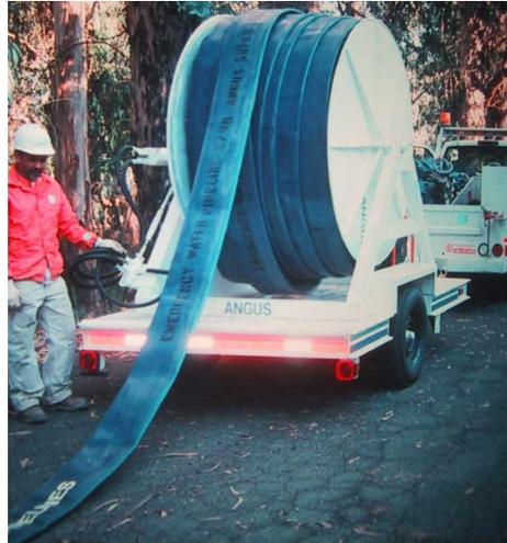
**Figure 6. Alternate Deployment of Flex Hose**
