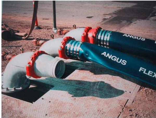
**Figure 3. Flex Hose Deployment in EBMUD System**
