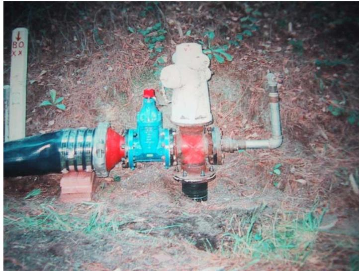
**Figure 4. Flex Hose Attachment To Fire Hydrant**
